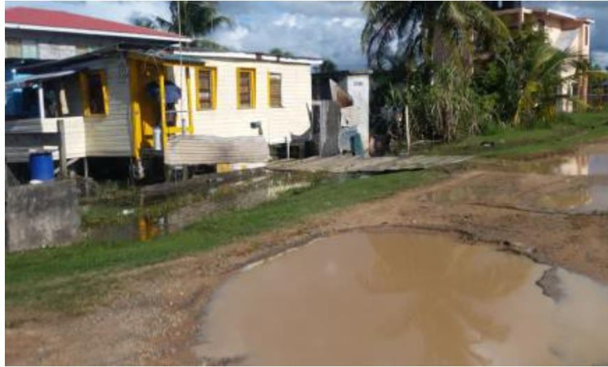
Figure 4-3: Potholed road in Sophia
