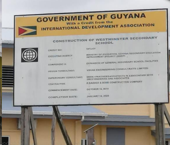
Figure 3-10: Secondary School under Construction
